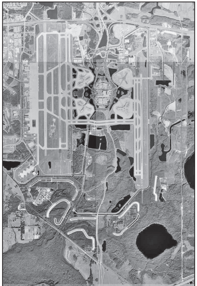
Photo E. Looking from above, here's a USGS digital picture of Orlando International Airport, Orange County, Florida. (Courtesy of USGS)
